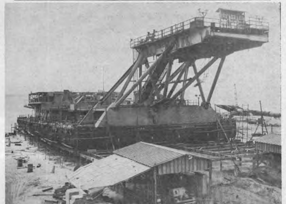
LARGEST UNIT WORKING ON LAKE MARACAIBO , Shell's G.P. No. 9 floating drilling barge and work-over rig, is hauled out at the Varadero Y Astillero del Zulia Compania Anonima, Maracaibo, Venezuela, shipyard for repairs. The unit was enlarged and the cantilever platform added in 1966 by the same shipyard. With the derrick and rotary removed, the barge, as shown, weighs 2,619 tons.
