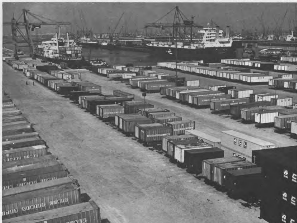
ROTTERDAM —A partial view of Europe Container Terminus (ECT) N.V.'s container terminal at Rotterdam's Prinses Margriethaven. Up to 2,000 forty-foot containers can be left at any one time in this 44-acre outdoor area. Atlantic Container Line, Hapag/Lloyd Container Line, Moore-McCormack Line, Sea-Land Service and United States Lines operate scheduled services to this ECT terminal. Two of the giant mobile container cranes available are shown.
