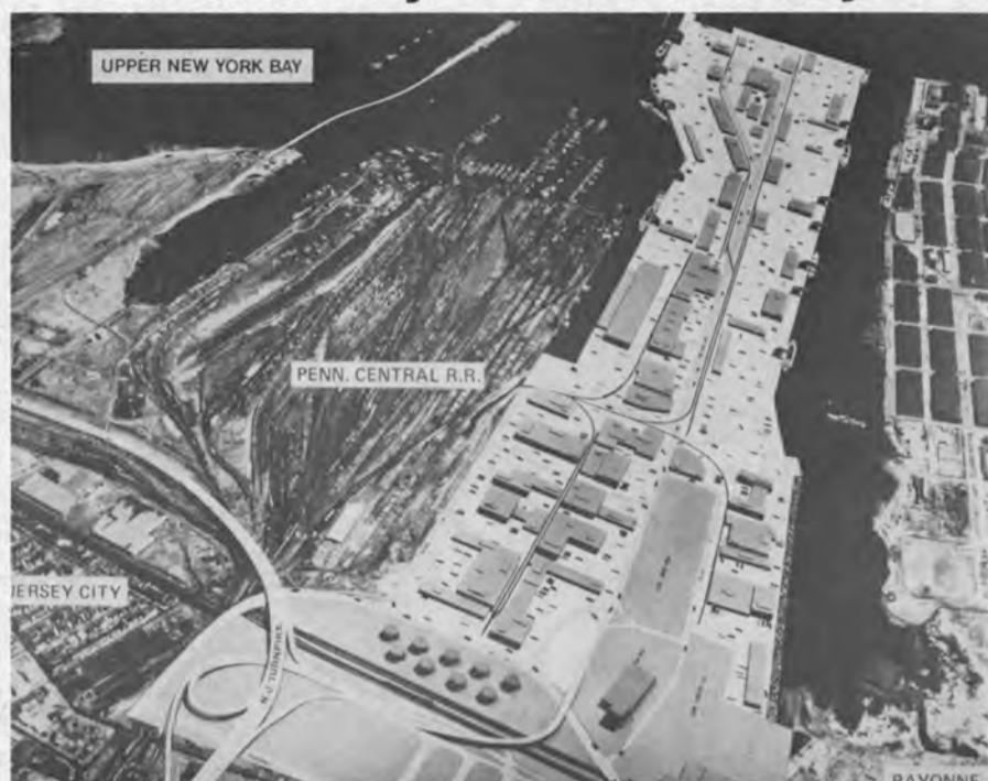
Model of Port Jersey superimposed on site. One-third of complex (foreground) will be 110-acre industrial center. Balance will be 300-acre deepwater port.
