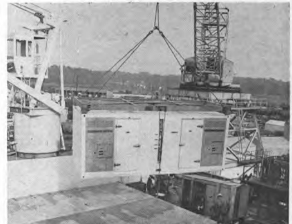
Loading of Dorsey refrigerated stores container equipped with Thermo-King units is tested at the shipyard. Stores containers are pre-loaded on the pier, thus reducing turn-around time of ship.
