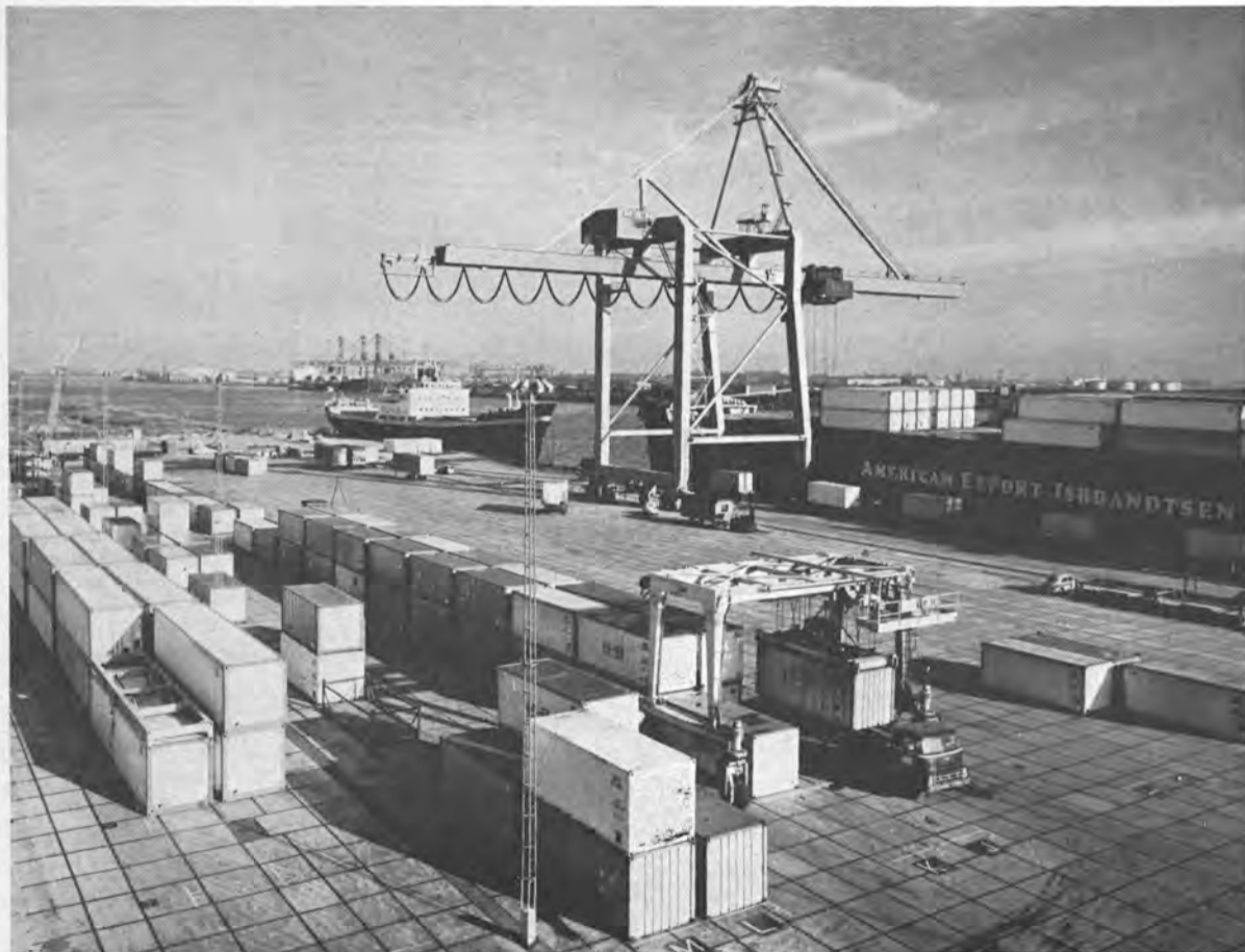
AMSTERDAM—Container Marine Lines, a subsidiary of American Export Isbrandtsen Lines, is one of the major users of Container Terminal "Amsterdam", a 164,000-square-foot facility able to accommodate 1,500 twenty-foot containers at one time. The crane shown has a 50-ton lifting capacity and an outreach of 118 feet over the water and 144 feet over the quay. This terminal also is the trans-shipment center for containers coming by rail to Amsterdam.
