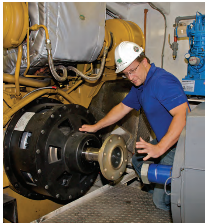
Installation of new hybrid equipment continues at Rainier Shipyard.
