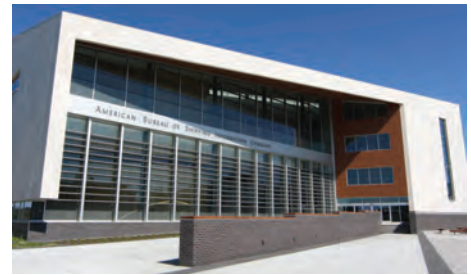
MMA's New Building, Simulator Facility.
