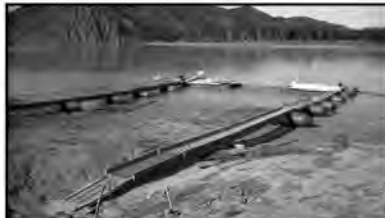
Floating dock and ramp assembly, Surplus Army "Bailey Bridge" style ramps and dock floatation system with custom steel ramps and floatation tanks
