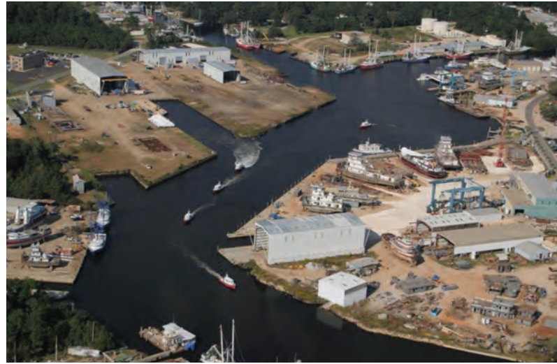
Aerial view of Horizon Shipbuilding's yard in Bayou La Batre, Ala. The new ferries will be constructed in the West Yard, visible in the upper right quadrant of the photo.
