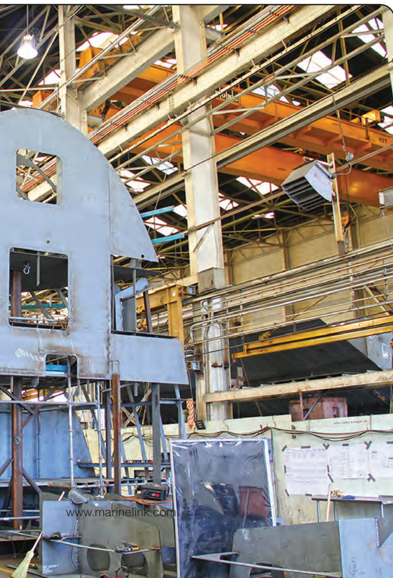
The fireboat under construction in Vigor's Seattle yard.
