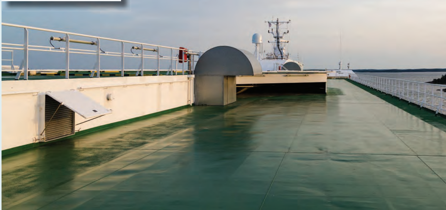
Air vents on the deck of a car ferry.
