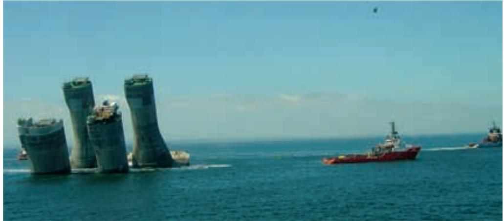
**Above: The tow out of concrete gravity base substructures (CGBS) for the Lunskeye A (LUN-A) and Piltun-Astokhskoye B (PA-B) platforms.**
