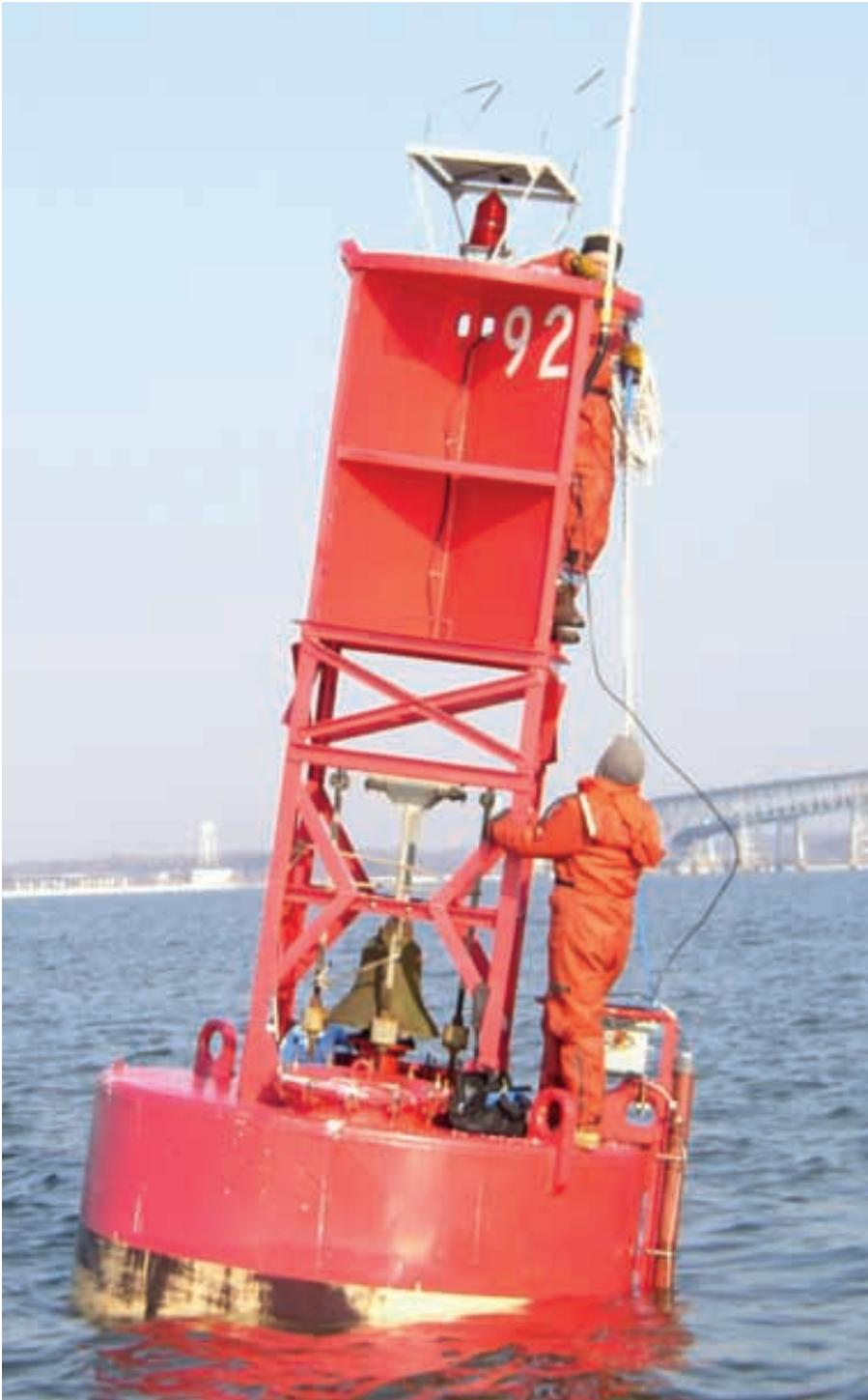
**NOAA Ports Technicians** at work installing a buoy-mounted current monitoring system in Chesapeake Bay.
