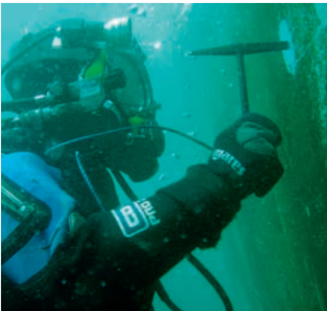
Cleaning the area before welding.
