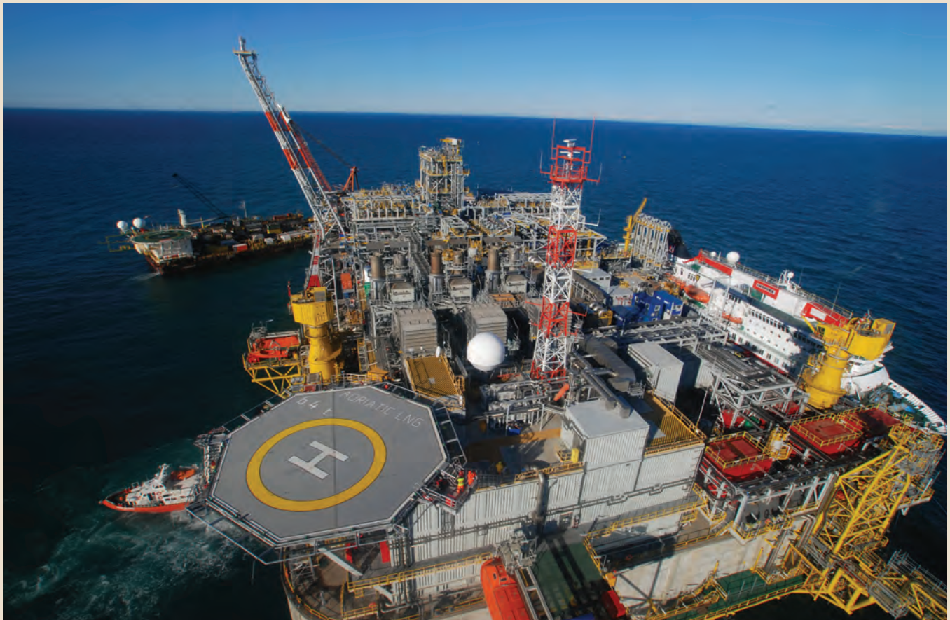
Adriatic LNG terminal – an example of multi-disciplinary services for one client
