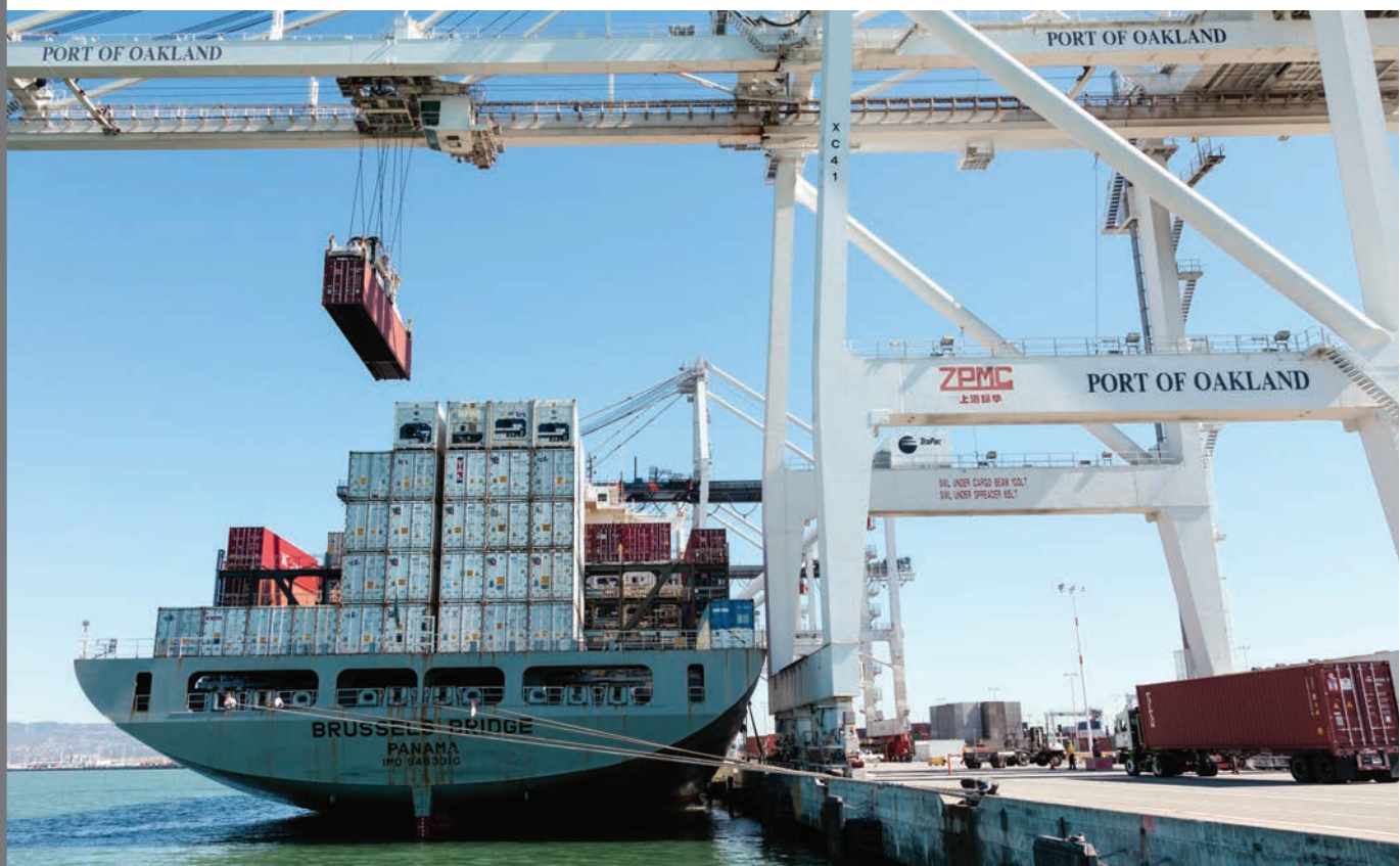
CREDIT: Port of Oakland
