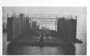
**NEW FLOATING DRYDOCK** put into operation by Martinolich Shipbuilding Corporation, Tacoma, Wash. The 1,250-ton lifting-capacity dock is provided with four centering posts controlled from the control tower, enabling the dockmaster to center the vessel quickly. The bilge blocks are attached to the centering posts and are cranked in from the vessel instead of the wingwall. The drydock is new in every respect and has been certificated by Philip F. Spaulding & Associates, Inc., of Seattle.
