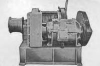
American Hoist and Derrick Company Winches with Westinghouse Motors, 50 HP, 230 Volts DC, complete with Con-tactor Panels, Master Switches, and Resistors.
