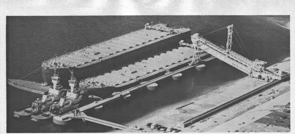
World's fastest phosphate loading terminal with 26,000-dwt barges and 5,000-hp tugs ready for service.
