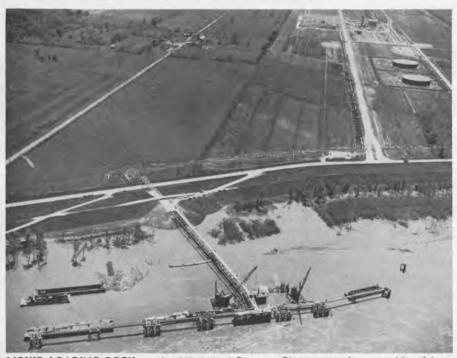
**LIQUID LOADING DOCK** on the Mississippi River at Plaquemine, La., capable of handling 95,000-dwt oceangoing ships is shown near completion in this aerial view. The 900-foot-long dock was built by Dravo Corporation, Pittsburgh, and will serve Hercules Incorporated's new methanol processing plant, shown in the right background.
