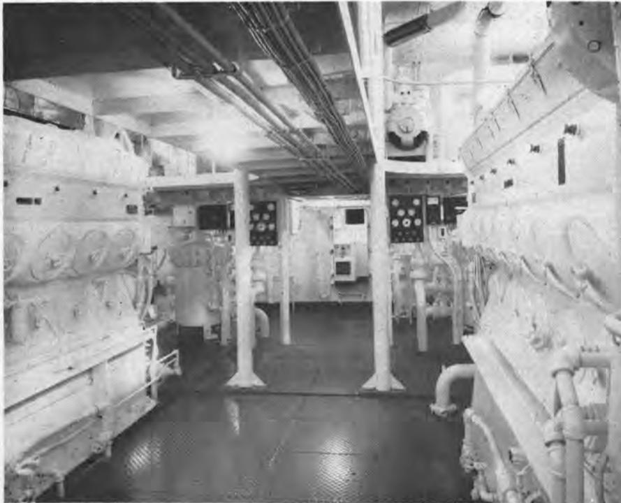
View down the centerline, looking forward, of the engine room showing the G-M diesels.
