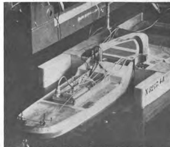
Tug and barge connected for model tests, showing barge wing walls and connection slots.
