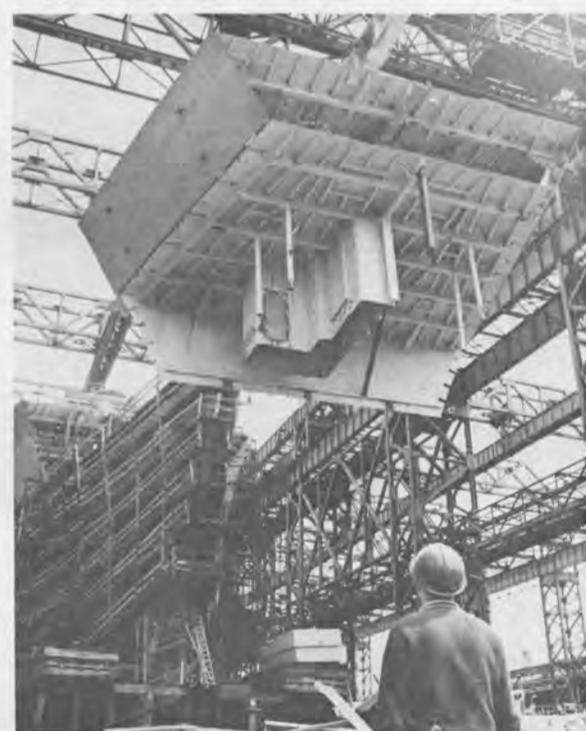
**HIGH RISE COMPARTMENT**—A rigger at the General Dynamics shipyard in Quincy, Mass., watches a 76-ton section being lifted nearly 100 feet to become part of the forward section of the United States Navy oiler-supply ship Kansas City, scheduled for launching this month. The 659-foot vessel, designed to provide operating forces at sea with rapid replenishment of fuel, ammunition, missiles and other supplies, is one of 14 surface ships to be built at the shipyard during the next three years.
