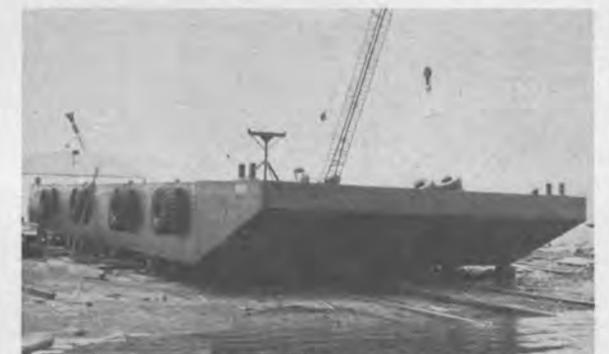
**DEEP-SEA DIVING BARGE LAUNCHED**—Jansen Marine Corporation, of Troutdale, Ore., recently launched a specially designed crane and deep-sea diving barge. The 155-foot by 60-foot by 12-foot steel barge will be outfitted with a 150-ton crane, winches, decompression chambers, helicopter port and complete living accommodations. The barge and her 20-man crew, will soon begin a six month tour of around-the-clock, deep-sea diving service in Alaska's Cook Inlet.
