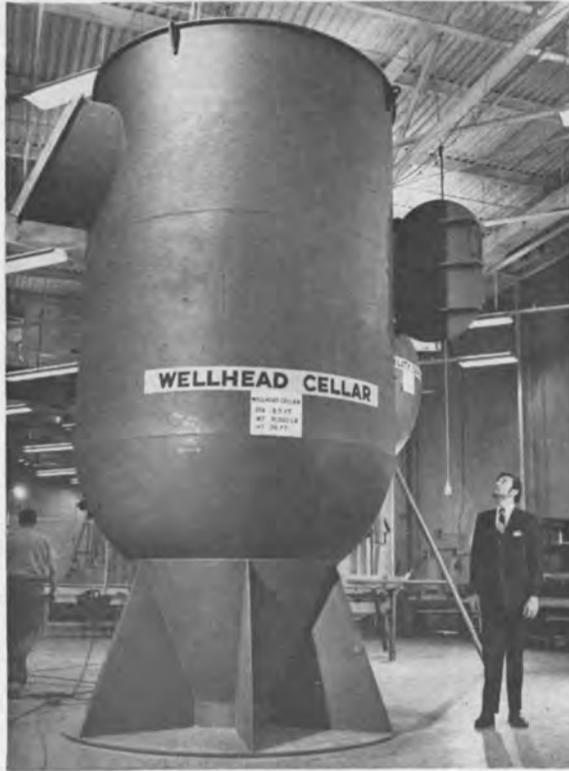
Mockup of wellhead cellar, part of Lockheed Missiles & Space Co. subsea petroleum system announced at Offshore Technology Conference in Houston, Texas. Lockheed system is for completion, production and maintenance of wells.
