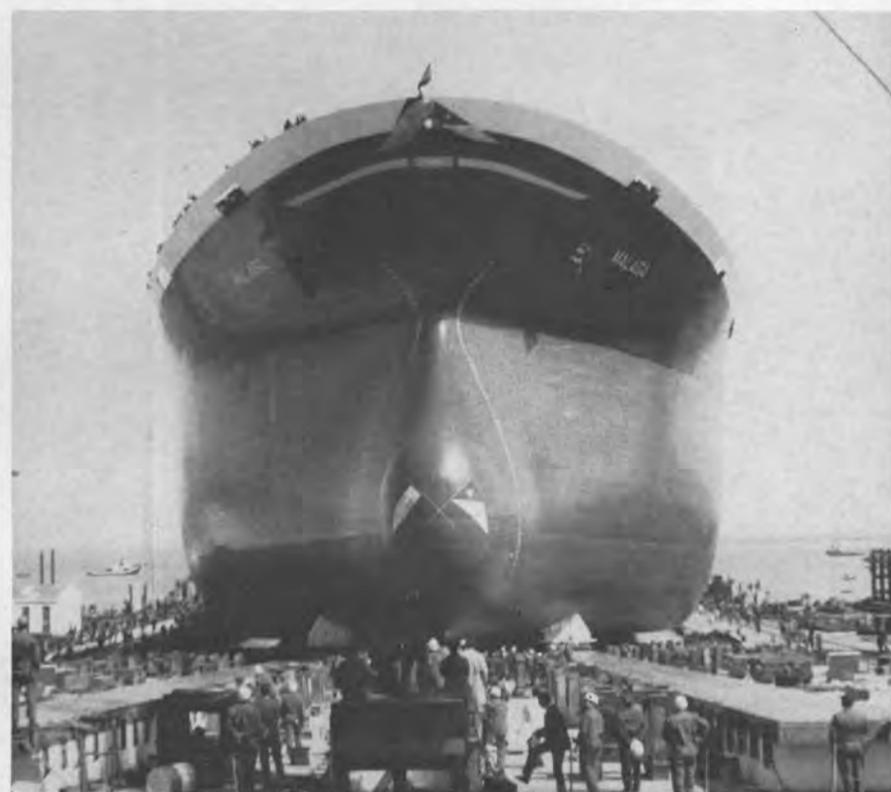
**LARGEST TANKER BUILT IN SPAIN** and the first of three 148,622-dwt ships was launched recently by Astilleros de Cadiz, S.A. The 944-foot 10½-inch Malago was ordered by Fletamentos Maritimos, S.A. The ship will be propelled by a Manises-Sulzer 12RD-90, 27,600-bhp diesel engine built by Astilleros de Cadiz. The yard has orders also for two 115,000-dwt and two 230,000-dwt tankers for foreign firms. The yard management also has announced plans to build tankers up to 330,000 dwt.
