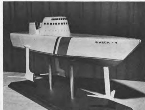
The ultra-high-performance hydrofoil designed by three students of the University of Michigan is capable of flying on its hydrofoils at 50 knots.
