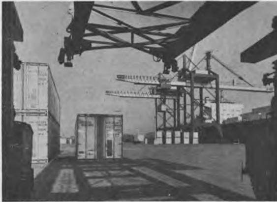
The Friedrich Kocks Company of Bremen, Germany, has been awarded an order for the construction and erection of four container transporters for the sea-wharf of Bremerhaven, Germany. Their design is similar to the one of the transporters previously supplied to the "Nordhafen" in Bremerhaven, shown in the photograph, however, having a capacity of 54 metric tons including spreader.
