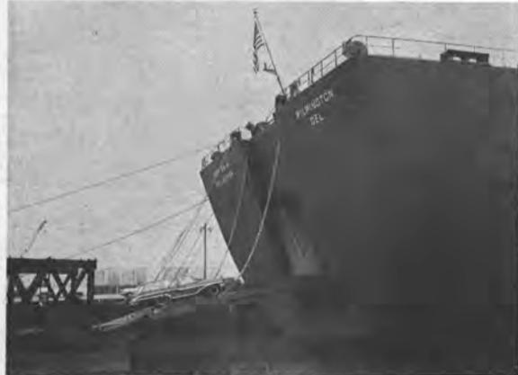
Adm. Wm. M. Callaghan loading cars over stern ramp from special facility developed by Northern Metal Co. which is still being utilized by MSTs.
