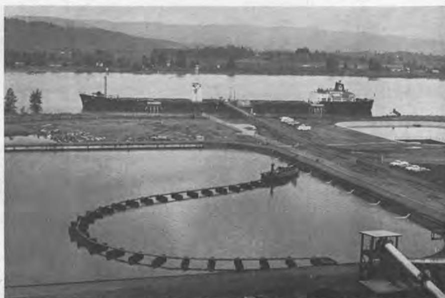
Thousands of tons of slurried iron ore are pumped from the SS Oread into storage pond at Oregon Steel Mills. Slurried ore is reclaimed by the dredge on the pond.
