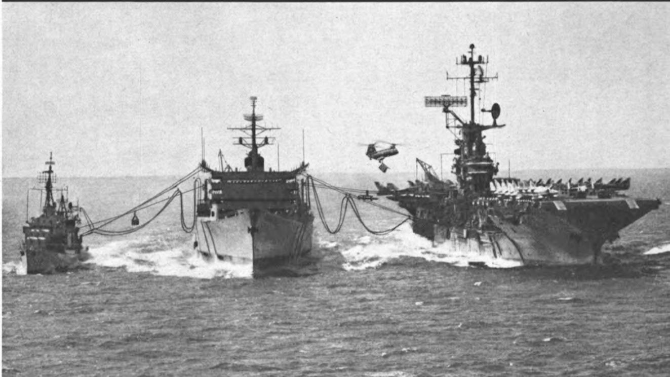
The U.S. Navy tackled a problem: how to transfer at sea the high volume of cargo needed for effective fleet operation. Through competitive bidding, Western Gear obtained contracts to turn a concept into working hardware.
