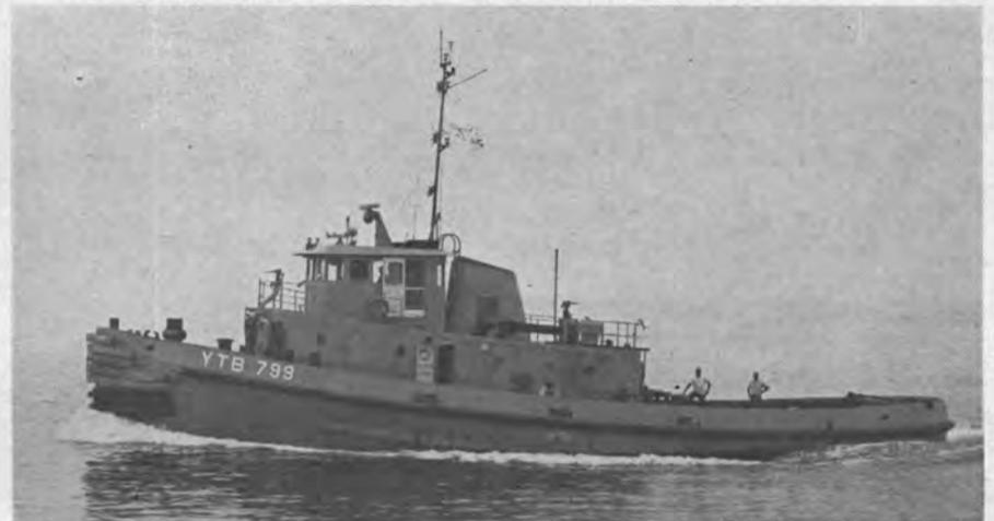
The U.S. Navy tug Natchitoches, first of four Navy tugs with automated engine rooms being constructed under a \$3-million contract with Southern Shipbuilding Corporation.
