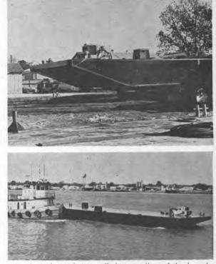
view shows barge being pulled over rollers of the launching system. Lower left photo shows the barge being tilted into the Atchofalaya Bay. The lower right view shows the barge retrieval after launching.
