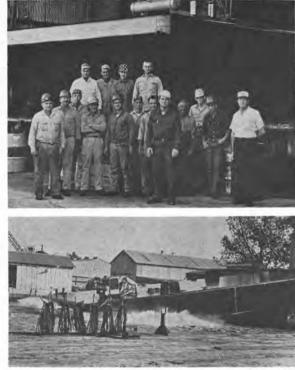
The above photo sequence indicates the unique tilttable launching system used by Conrad Industries of Morgan City, La. The ARC-23, a 120-foot by 30-foot by 7-foot-3-inch barge built for A. R. Crane Jr., was constructed inside the fabrication building. Upper left photo shows part of the yard force which built the barge with Parker Conrad (far right), president of Conrad Industries, and Frank Elliot (center foreground), barge building superintendent, prior to launching. Upper right
