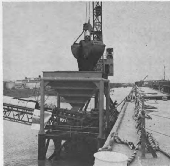
A view of crane offloading barges in Harvey, La., and depositing raw material on conveyor belt.
