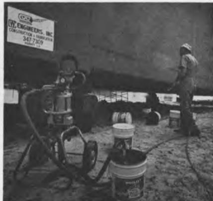
A barge in Harvey, La., being coated with 98 percent solids glass-filled polyester resins using a Spee-Flo Commander Special model.
