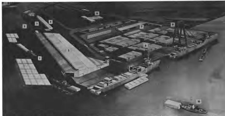
Artist's rendering of the world's first LASH terminal being built in San Francisco for Pacific Far East Line. This view shows: 1. lighter storage basin, 2. two heavy-lift cranes of 50-ton capacity each, 3. lighter maintenance yard, 4. service building, 5. lighter freight station, 6. administration building, 7. container freight station, 8. container yard, 9. container crane, and 10. tug pushing seaworthy lighter. Cost of terminal is \$21.5 million.
