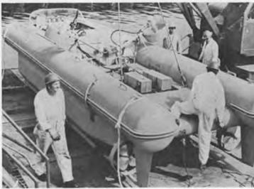
The catamaran-type hulls on the vehicle are fabricated of ASTM A36 steel plate of 26-inch diameter.
