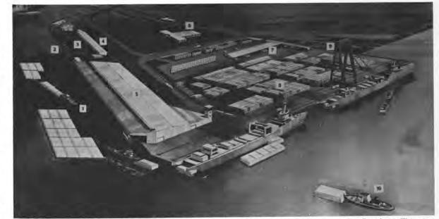
Artist's rendering of the world's first LASH terminal being built in San Francisco for Pacific Far East Line. This view shows: 1. lighter storage basin, 2. two heavy-lift cranes of 50-ton capacity each, 3. lighter maintenance yard, 4. service building, 5. lighter freight station, 6. administration building, 7. container freight station, 8. container yard, 9. container crane, and 10. tug pushing seaworthy lighter. Cost of terminal is \$21.5 million
