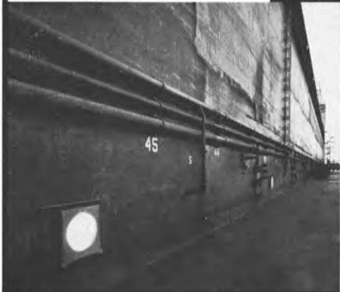
Services include compressed air, oxygen, acetylene, steam, salt and fresh water, sewage lines, AC/DC power, P.A. and phone circuits—all with numerous outlets. Strong lighting is provided throughout.
