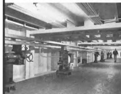
Spacious safety decks at the 68-ft level in both wingwalls house the pumps, motors, substations, and other equipment. They are compartmented by watertight bulkheads.
