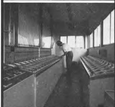
Control of pumps and flooding for all 40 ballast compartments through banks of buttons and indicators is centered here in the control house atop the west wingwall.
