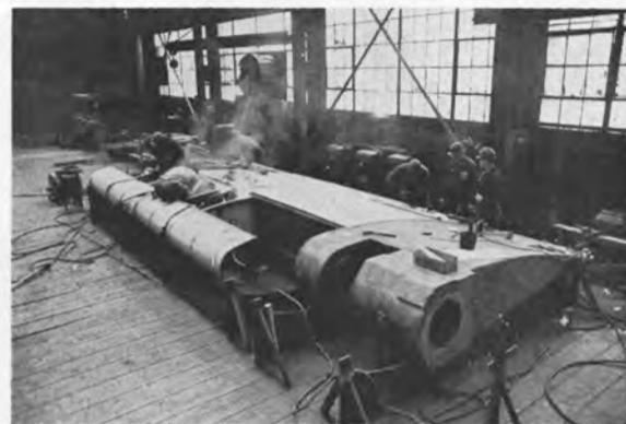
Craftsmen of Bethlehem Steel's Hoboken, N.J., ship repair yard rebuilding the rudder for the 28,000-dwt tanker *S/S Eagle Courier*.
