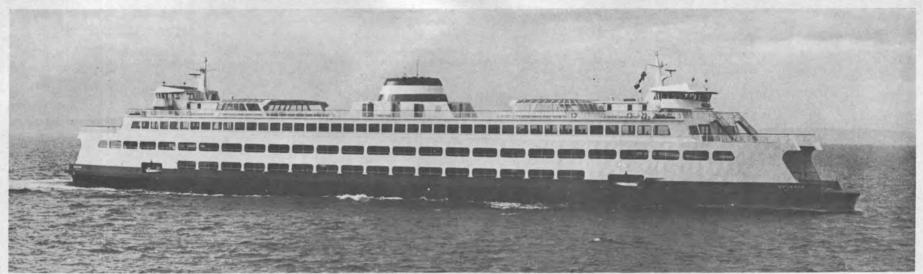
Powered by General Motors Electro Motive Division 8,500-hp diesels driving Coolidge propellers, the double-ended Spokane had to go through two complete trial tests—once for each end.
