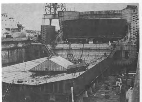
JOINING OPERATION in the ship requires careful planning and manufacturing of the tank segments. This view shows the inner bottom which serves as a jig for assembly.
