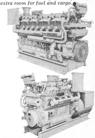
Cat Electric Sets. Available in 40 to 900 KW configurations. Handle auxiliary and emergency needs above or below deck.
