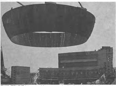
TANK SEGMENT being moved by cranes to the ship for joining with a lower section. Some shipyards will assemble tanks completely prior to installation aboard the ship.
