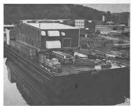
Shown on a barge is one of five sections of the B.P. Alaska, Inc. base operations camp that will be carried to Alaska's North Slope. In the background are four sections of the camp yet to be loaded.
