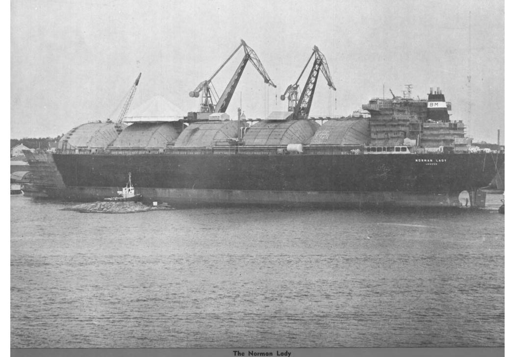
Rosenberg Verft, Stavanger, Norway **Launches First LNG Carrier Utilizing** The Moss Rosenberg Tank System
