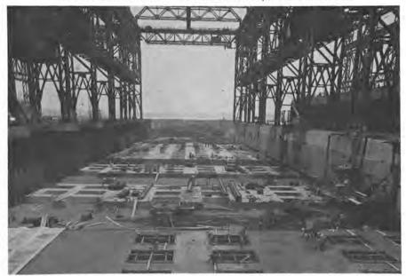
Workmen are nearing completion of the concrete slab floor on Building Basin Twelve at General Dynamics, Quincy Shipbuilding Division. The Basin will be the site of the first liquefied natural gas tanker to be constructed in the United States.
