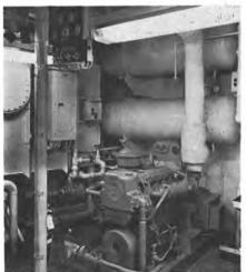
Detroit Diesels drive the Delco generators for electric power.
