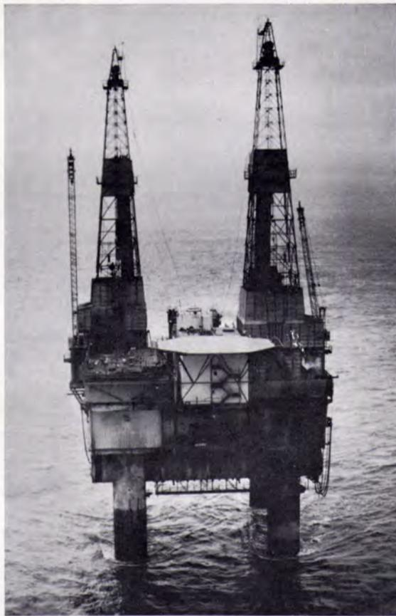
This production platform in Cook Inlet, Alaska, represents a complete oil field operation, including water injection field. Johnston pumps, highly suitable because of their vertical configuration, serve as crude oil loading pumps.
