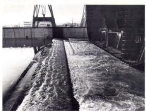
As the repair dock floods, the water flows over the sill into the newbuilding section to float the ship.
