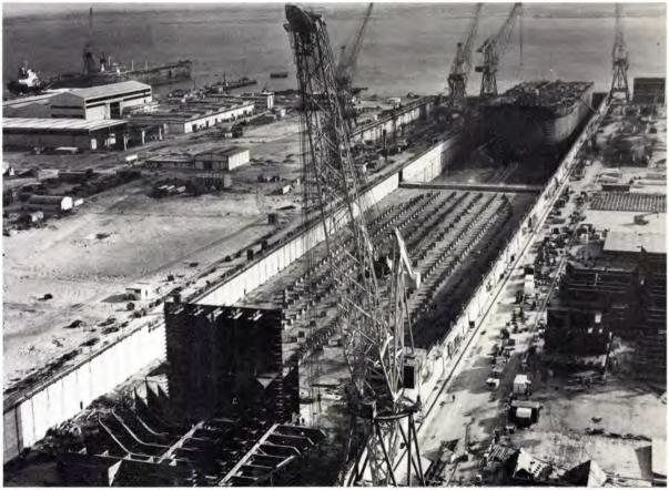
Overall view of the 1,378-foot-long building platform, foreground, with structure being erected for a 316,000-dwt VLCC and the 1,476-foot-long drydock with the 878-foot tanker forebody in it after being floated.
