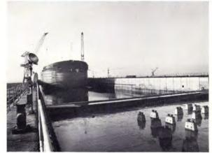
This view shows the hull section after being floated into the drydock and the dock being pumped.
