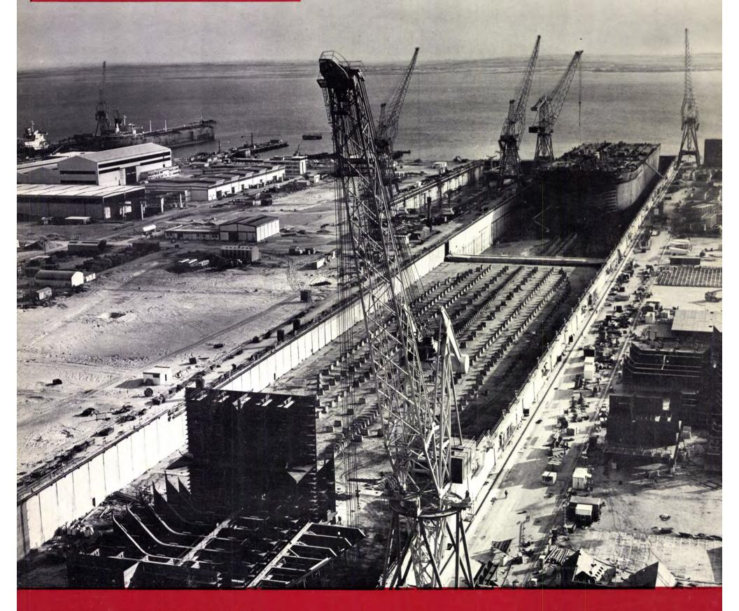
New Setenave Yard Is Building Ships On Dry Land And Floating Into Graving Dock For Launching
