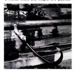
One of the Aero-Casters in position and under water pressure is shown between concrete runway and ship cradle.
