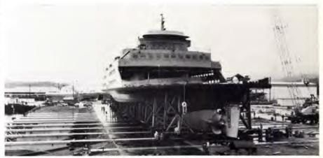
The 3,500-ton ferry, Queen of Alberni, is shown being positioned on launching ways by using the Aero-Caster System, developed by Aero-Go, Inc.
