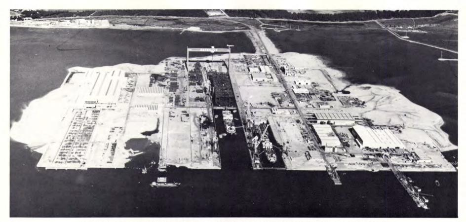
Setenave Shipyards, built on man-made island in the Sado River, can build and repair ships up to 700,000 dwt.
