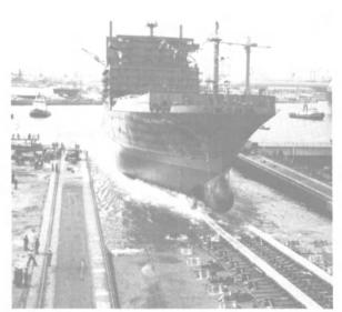
**I.AUNCH IN FRANCE** — Hull No. 308, the **Ro-Ro Manhattan**, was launched recently at the French shipyard Chantiers de France-Dunkerque. The 12,640-dwt ship has a length of 170 meters and beam of 25 meters (558 by 82 feet). She is designed to carry containers, trailers, platforms, motor cars, and heavy lifts loaded as roll-on/roll-off cargoes. She will carry 684 TEUs. The ship was ordered by a subsidiary of the shipbuilder, Societe Dunkerquoise d'Armement.
