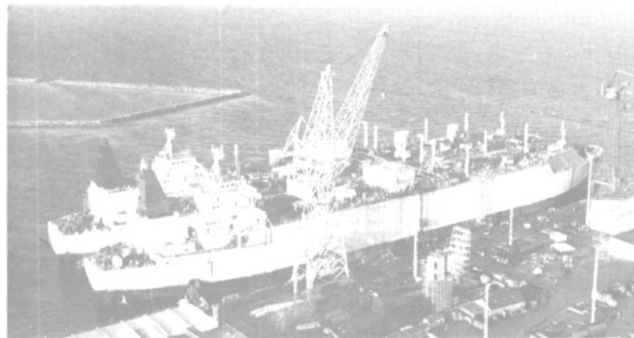
One of these two 133,000-cubic-meter LNG carriers undergoing final outfitting at the Kockums yard in Sweden has been sold to a West German consortium. The Malmo yard has also granted an option on the second ship.
