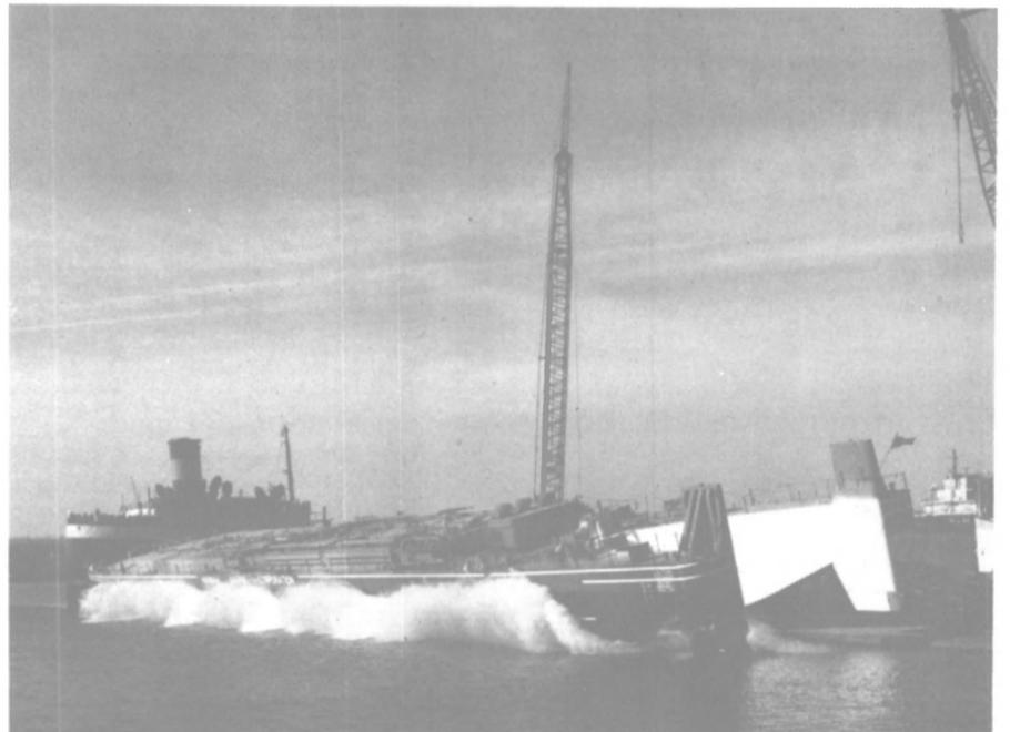
Tank barge Hannah 6301 makes big splash in Lake Michigan during recent launching at Bay Shipbuilding's Sturgeon Bay, Wis., yard. With a capacity of 63,000 barrels, the 407-foot vessel is largest in nine-barge fleet of Hannah Marine Corporation.
