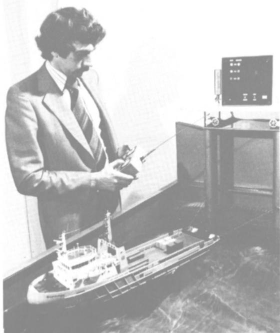
A new, unique mooring system that will keep a supply vessel permanently and safely moored to an oil rig at a pre-determined distance even in the worst sea conditions encountered in the North Sea is being developed in Scotland. A model of the Scomag Hydraulics Ltd. system is shown above being tested in the company's factory at Bellshill, Lanarkshire.
