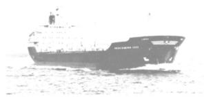
The 17,780-dwt products carrier Pertamina 1023 (shown above), constructed at the Maizuru Works of Hitachi Zosen, was delivered recently to Scorpa Pranedya Shipping, Inc., Panama. She is the fifth products carrier of the same type to be delivered by Hitachi for the transportation of refined pe-
