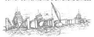
3500 Ton Dock 200' x 100' 90' Between Wing Walls 1500 Ton Dock 160' x 80' 70' Between Wing Walls 850 Ton Dock 60' x 150' 50' Between Wing Walls 300 Ton Dock 50' x 80' 40' Between Wing Walls
