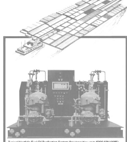
Typical Westfalia Fuel Oil Purification System (for viscosities up to 6000 SRI/100°F). Centri-Pack module incorporates two OSA self-cleaning Oil Purifiers.
