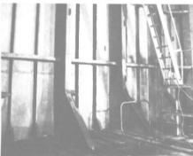
Shown here after three years of user-trial service on Rowbotham Tankships' products carrier Echoman, the Amercoat 346 lining is in very good condition.
