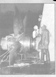
Our propeller shaft seals SPLITEX and MONEX, for shaft diameter 100 mm to 1200 mm, were introduced in 1985. Within the first years of manufacture they have exceeded all expectations with regard to the number of installations carried out.
