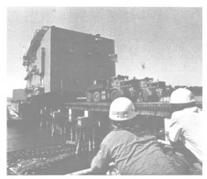
LARGEST OIL MODULE EVER built for ARCO Alaska, Inc., is loaded onto a Crowley Navigation barge positioned on Drydock 4 at Portland Ship Repair Yard (PSRY) for ship-ment to Alaska's Prudhoe Bay. One of eight modules fabricated at PSRY for ARCO by Wright Schuchart Harbor Co., the two largest are 3,200-ton turbine compressor modules. The 11-month, \$40-million project generated peak employment for 1,600 workers.
