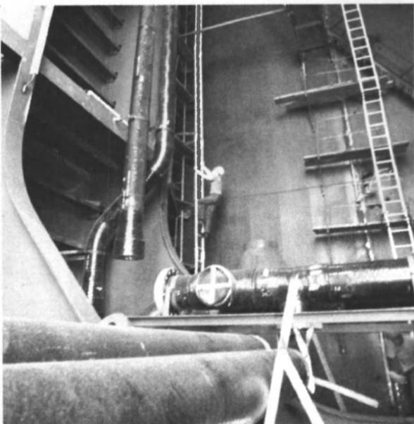
Bondstrand Series 2000M is used for a host of applications including in-tank ballast lines. Series 2000M is designed with extra-heavy walls to withstand external pressures when operating at full vacuum inside large tankers.
