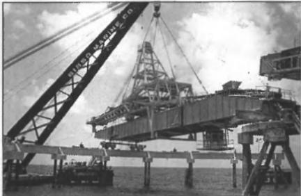
A Bisso Marine derrick repositions a 220-ton ship loading conveyor on its pivotal foundation.
