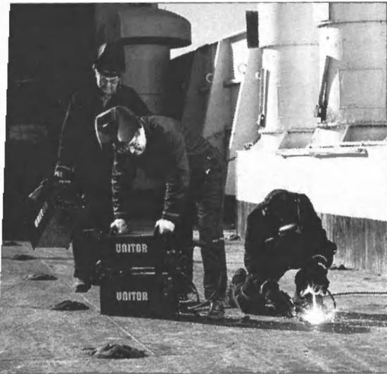
Unitor introduced a compact, lightweight, multipurpose electric welding unit for shipboard use. Developed with Lincoln Electric, the UWI-350MP is designed to cover all shipboard arc welding and cutting requirements — but for operators who only require conventional coated electrode welding, comes in a basic form with a comprehensive list of “add-on” features.
