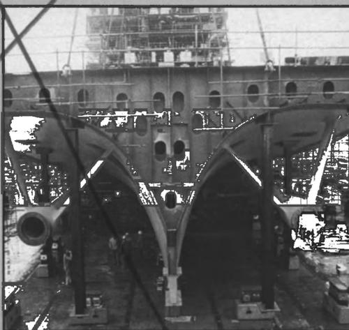
Shipyard photo of Veendam's propeller supports.
