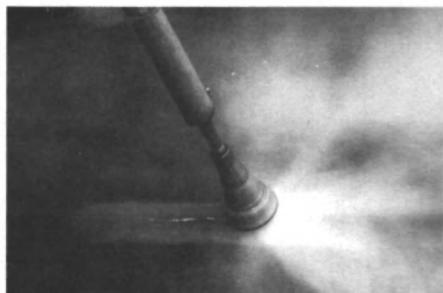
High-pressure waterblasting produces a clean surface in minutes.
