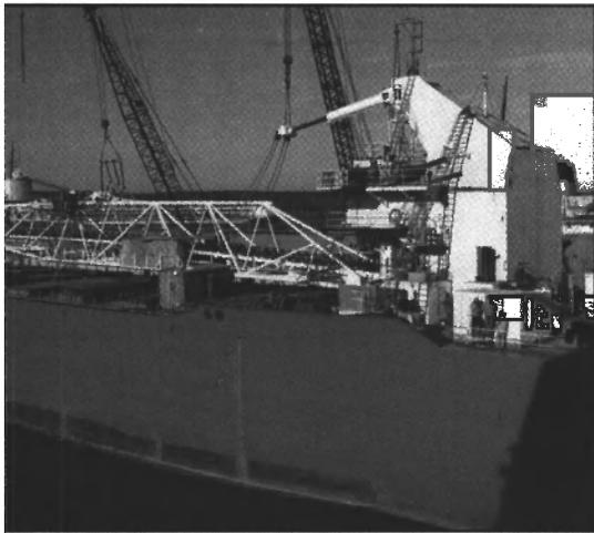
**Top:** View from stern of *Pathfinder*, a tug-barge undergoing conversion at Bay Shipbuilding, shows support structure for boom at right, with hydraulic cylinder being installed.
