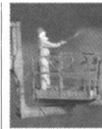
During the Dubai dry-docking, Sea World's 30 cargo tanks were coated with Sigmaguard CSF, a coating specifically designed to protect cargo tank bottoms.
