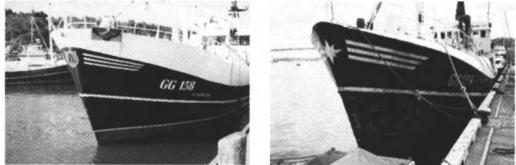
(Left above) 'Sunnanland' – virtually free of corrosion after 2 years in service working in ice. The hull is protected with 2 coats of Jotamastic 87 and Seavictor Antifouling. The only maintenance required was fresh water cleaning, blastcleaning slipway support marks and application of 1 gallon of Jotamastic 87!
