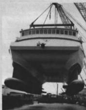
Built in 1996 for the Monterey Bay Aquarium Research Institute by SWATH Ocean Systems, the twin-hulled vessel measures 117 x 53 ft. (35.6 x 16 m) with a displacement of 419 long tons.
