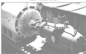
2 Fuel Oil Transfer Pumps Size 8x6 Mfg: DeLaval 700/525/350/250GPM@150psi Horizontal Model A32NX437 Motor: Continental 100/75/50/37.5HP 440/3/60 TEFC
