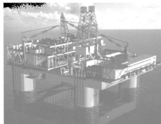
will be produced using the "Thunder Horse PDQ" platform. Displacing 129,000 tons, this will be the largest semi-submersible production platform in the world. It will be delivered from Korea in 2004.
