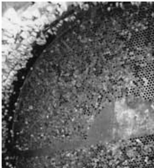
Typical fouled condenser tube plate.
