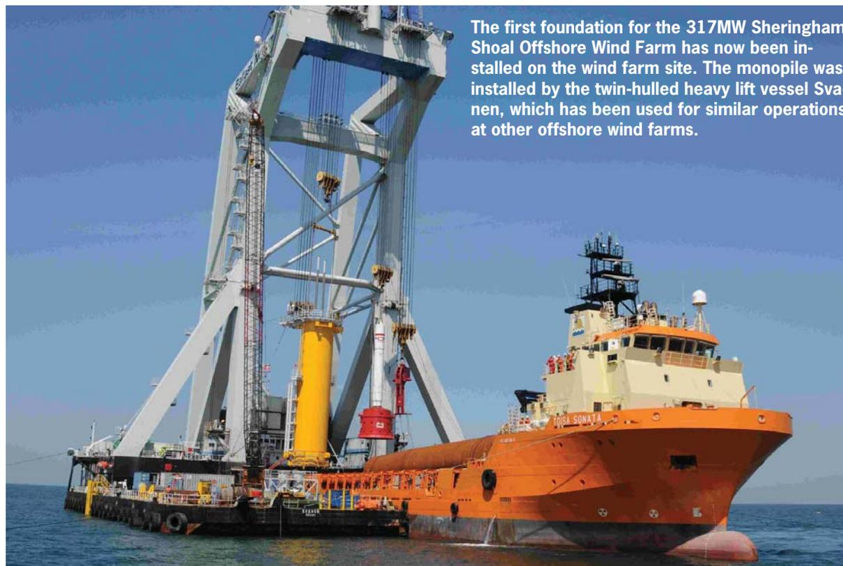
The first foundation for the 317MW Sheringham Shoal Offshore Wind Farm has now been installed on the wind farm site. The monopile was installed by the twin-hulled heavy lift vessel Svanen, which has been used for similar operations at other offshore wind farms.
