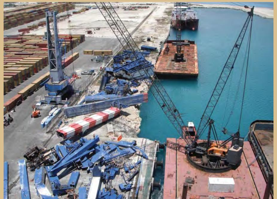
**Mobro ABS barge mounted Ringhorse and American 11320 (450t) crawler lifts collapsed container crane from water in Freeport, Grand Bahama.**
