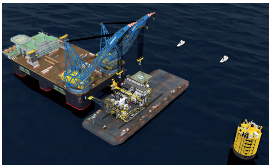
Figure 2. Installing Gulfstar FPS triple-deck topsides onto spar.
