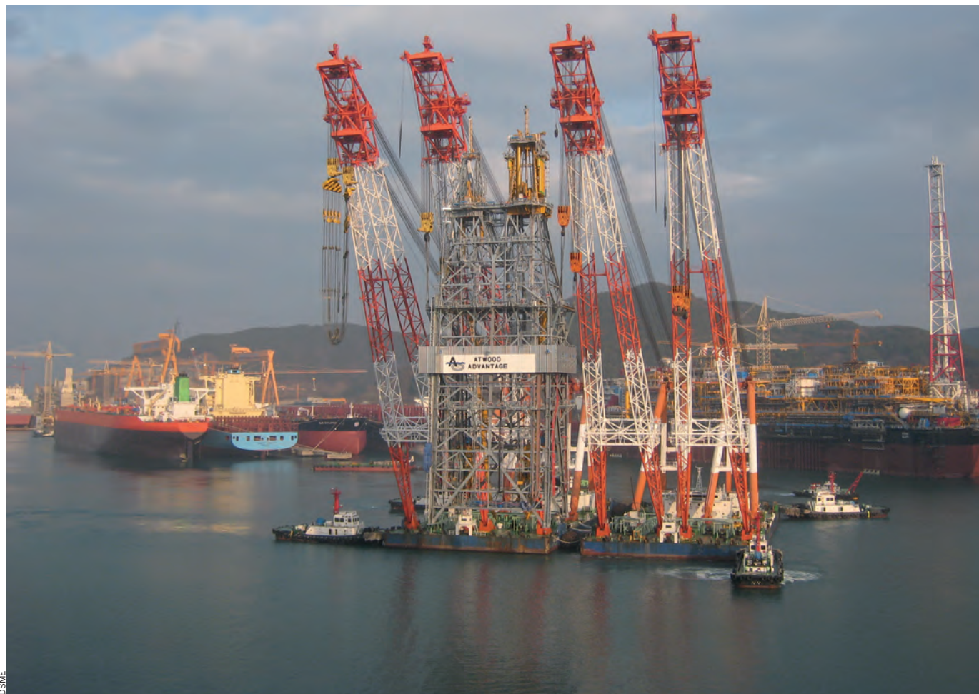
Two derrick barges move the Atwood Advantage 's drilling derrick into place.
