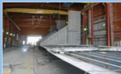
START OF CONSTRUCTION 5,000 CU.YD. SPLIT HOPPER DUMP SCOW
