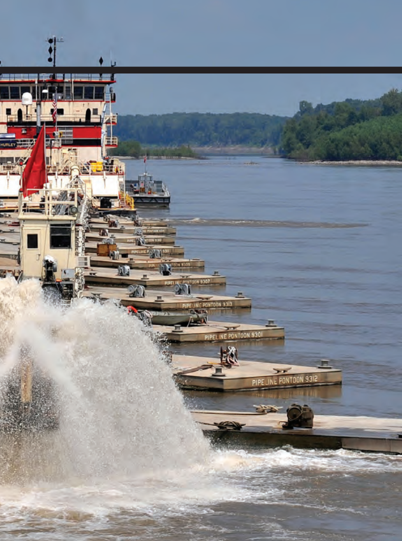
USACE Dredge Hurley In operation on the Mississippi River.
