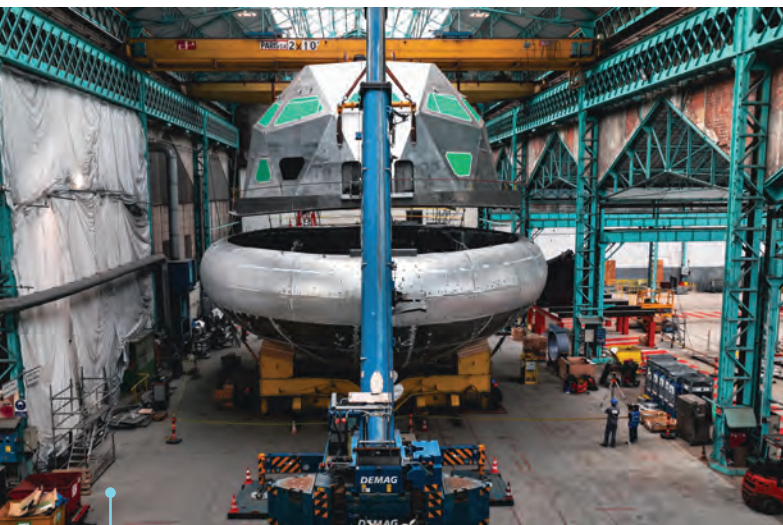
The Tara Polar Station under construction.
